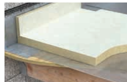
Typical Installation - Timber Deck
